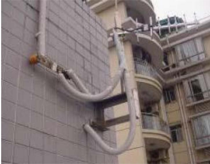
Cable layout through walls – “U” Dripping bend
